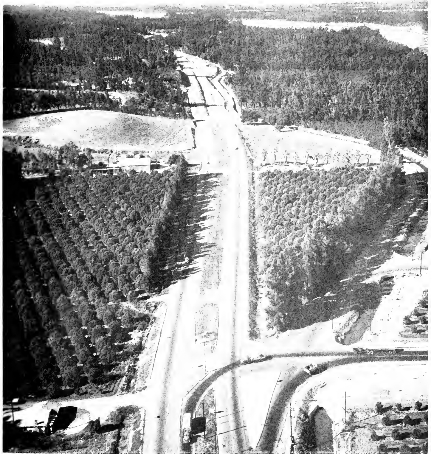
Looking westerly along the Santa Ana Canyon Freeway, showing in foreground junction with Yorba Boulevard. Santa Ana River in background.
